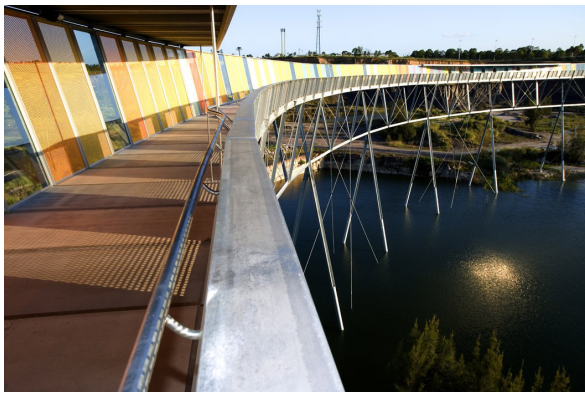
The Ring Walk, an aerial walkway and outdoor exhibition space, twenty metres above the brick pit floor, gives a former brick pit a genuine urban connection and presence within Sydney's Olympic Park in Australia. The ring walk facilitates both access and interpretation to the brick pit, while fully recognizing its extremely fragile habitat. (Project by Durboch Block Architects)
