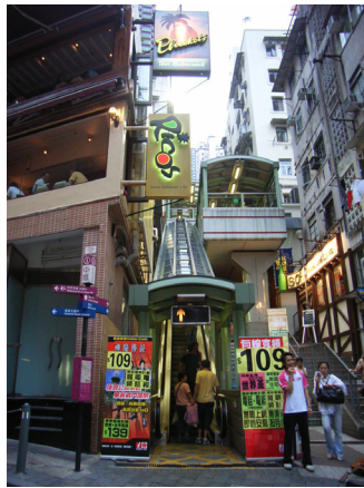
Mechanical stairs in Hong Kong, China, turn into a place of consumption and a residence.
