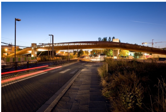
The footbridge in Villetaneuse, France, is an intrinsic junction of larger units of public uses and joins two groups of university buildings, turning the connection into a gathering place (Project by DVVD).
