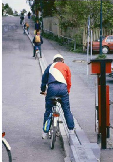
The Trampe Bicycle lift in Trondheim, Norway.
