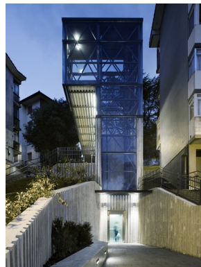
An outdoor elevator connects the mountainside neighbourhoods of the Spanish town of Errenteria, Spain, to those in the valley (Project by Vaum).
