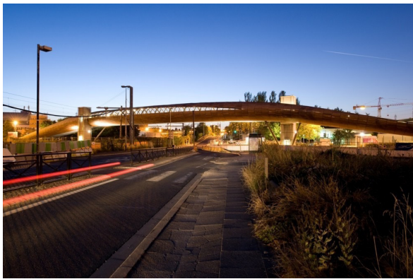
The elevated bicycle roundabout safeguards bikers from the busy thoroughfare in Eindhoven, the Netherlands (Project by IPV Delft).
