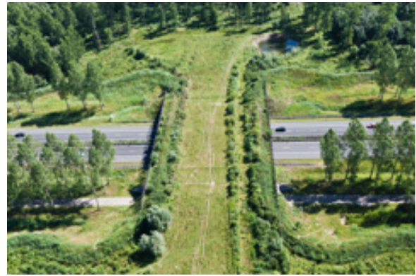
The ecoduct guarantees a safe passage for wildlife, high above car traffic on the A2 in the Netherlands.
