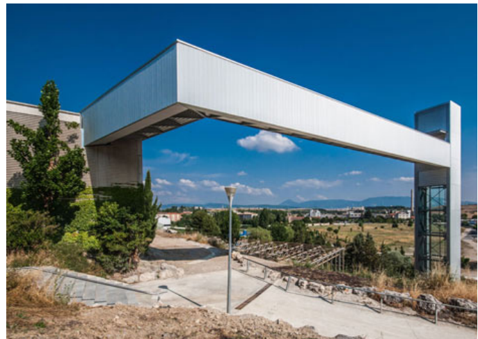
A footbridge with an urban elevator in Echavacoiz Norte, Pamplona, Spain, creates a clear marking figure in the urban panorama (Project by AH Asociados).
